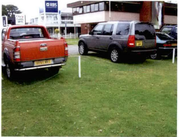
The above image shows the grid force system with grass growing through, this has been installed for approximately two months with the grass now strongly visible
